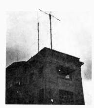
Roof-top antennas (above) are smaller and lighter than those used for transmissions on the 2-mc. band. The VHF antenna can be made extremely directional to eliminate interference, increase pickup from low-power transceivers while listening and increase the e.r.p. (effective radiated power) when transmitting. A typical control-tower operating position is shown at top-right and a scale-model canal plotting board setup is shown at right.
