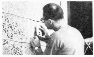
and cut-out the opening with a saber or keyhole saw. If your home is brick faced mount a waterproof electrical box on the brick and mount the remote in the box—most outdoor remote units have rubber seals for weatherproofing.
